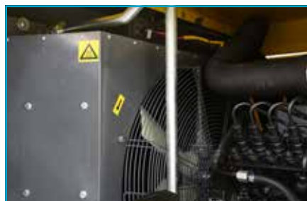
Enhanced cooling system for 50°C high ambient temperatures.
